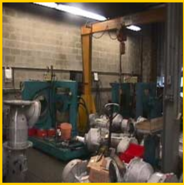
A Section of the Transmission Shop
