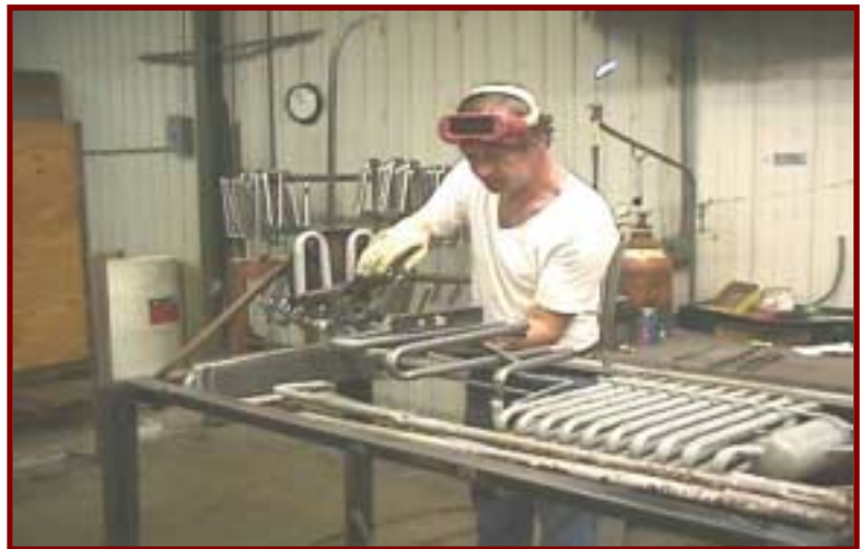
The new evaporator is welded in place
